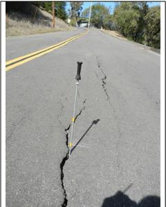
Circle Oaks Drive (COD) has some very significant fractures and cracks that extend several feet into the sub grade and also has obvious subsidence in these same areas. And since the cracks are open and clean, they are recent. In the above right hand photo notice curb movement. Left photo shows a ¾" probe that is 22" into a crack.
